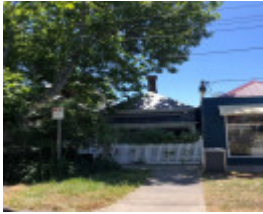
41 Union Street, Armadale
