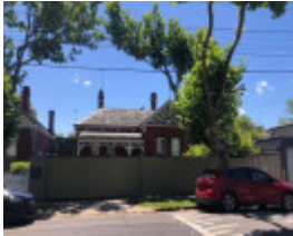
51 Union Street, Armadale
