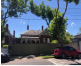
51 Union Street, Armadale
