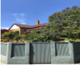
53 Union Street, Armadale
