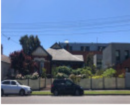
55 Union Street, Armadale
