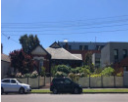
55 Union Street, Armadale
