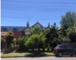
61 Union Street, Armadale
