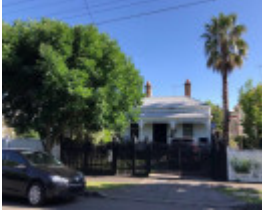
13 Barkly Avenue, Armadale
