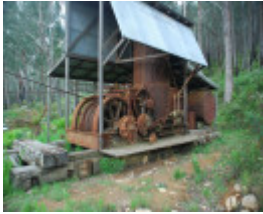
WASHINGTON WINCH SOHE 2008
