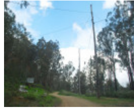
WASHINGTON WINCH SOHE 2008
