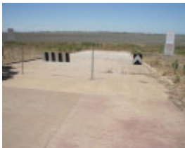
H2208 Boga Slipway Feb 09 PM2
