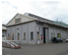
Before Photograph - Reference F3916 2014
