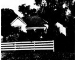
93 - House 780 Heidelberg Kinglake Rd - Shire of Eltham Heritage Study 1992
