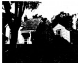
93 - House 780 Heidelberg Kinglake Rd_02 - Shire of Eltham Heritage Study 1992
