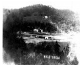
94 - Railways Residence Palm Cypress Trees Hurstbridge_02 - Old photography presumably taken in or soon after 1912 showing the Hurstbridge Railway Station and on the right hand side this house, which predates all of the nearby buildings (ELHPC No.1004) -
