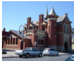
H1462 Bairnsdale Court House from the SW
