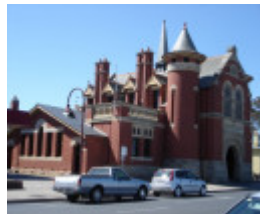
H1462 Bairnsdale Court House from the SW
