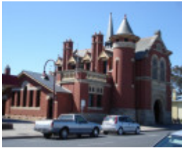
H1462 Bairnsdale Court House from the SW
