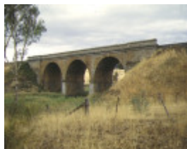
1 harcourt railway precinct harcourt side view apr1998
