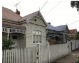
Dudley Street Precinct - 37- 45 King Street
