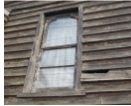
Church (former), 170 Albert St Brunswick
