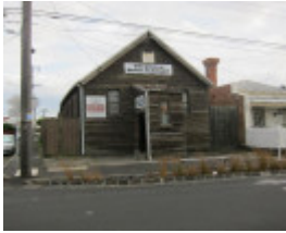
Church (former), 170 Albert St Brunswick
