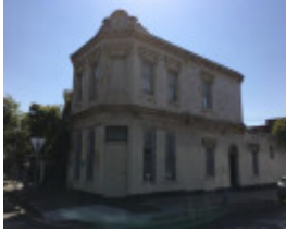
Shop - 209 Barkly Street
