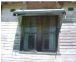
H01832 thologolong homestead window detail mar02 pm1
