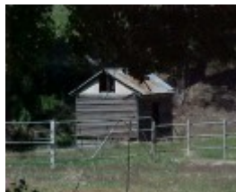
H01832 thologolong homestead workman s hut mar02 pm1
