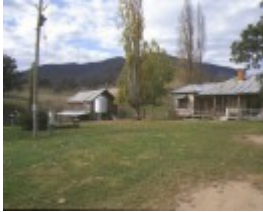
1 thologolong homestead walwa may99 pm1 general view
