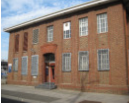
Telephone Exchange - 3-5 Frith Street, Brunswick
