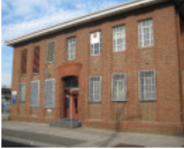
Telephone Exchange - 3-5 Frith Street, Brunswick
