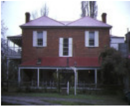
gundowring homestead gundowring rear view
