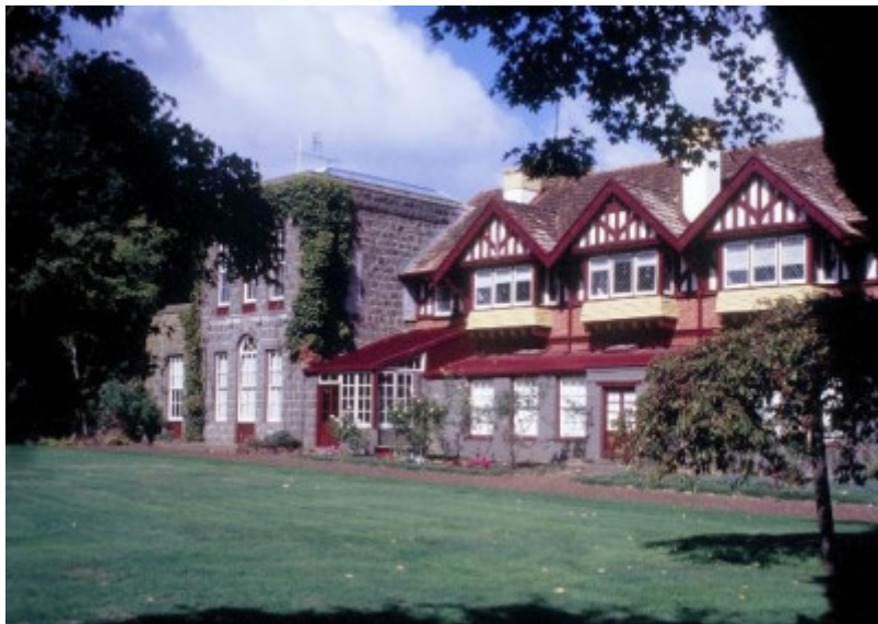
h00289 1 murndal murndal road hamilton homestead
