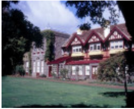
h00289 1 murndal murndal road hamilton homestead
