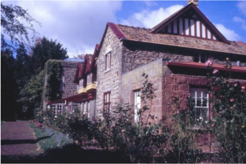
h00289 murndal murndal road hamilton homestead close up
