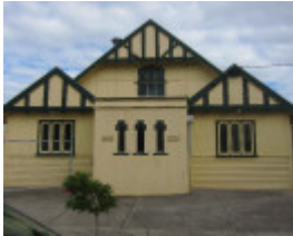
Church, 384 Moreland Rd Brunswick West
