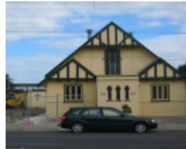
Church, 384 Moreland Rd Brunswick West
