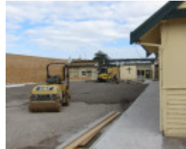
Church, 384 Moreland Rd Brunswick West
