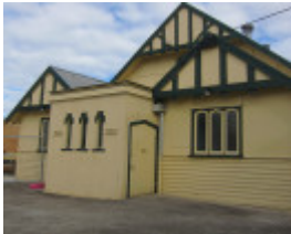
Church, 384 Moreland Rd Brunswick West
