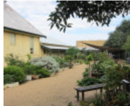
Church, 384 Moreland Rd Brunswick West
