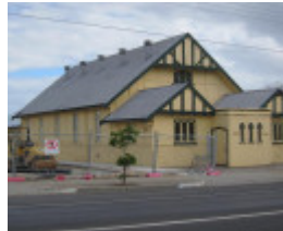
Church, 384 Moreland Rd Brunswick West
