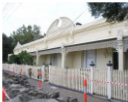
QUEENS TERRACE SOHE 2008
