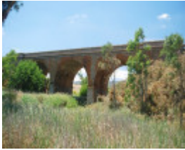
RAIL BRIDGE SOHE 2008
