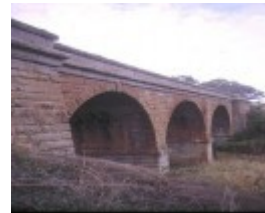
1 rail bridge over barkers creek harcourt side elevation apr1995
