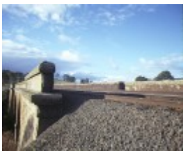
rail bridge over barkers creek harcourt railway tracks & siding aug1984
