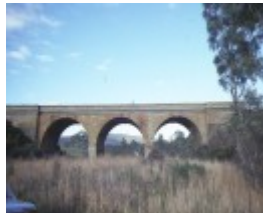
rail bridge over barkers creek harcourt side view aug1984
