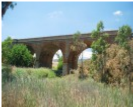
RAIL BRIDGE SOHE 2008
