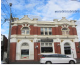
State Savings Bank of Victoria, 840 Sydney Rd Brunswick
