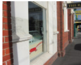
State Savings Bank of Victoria, 840 Sydney Rd Brunswick
