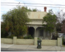
House - 232 Victoria Street, Brunswick
