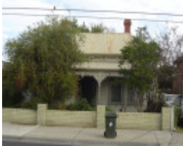
House - 232 Victoria Street, Brunswick
