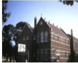
primary school number 1467 malvern road hawthorn rear view 1994
