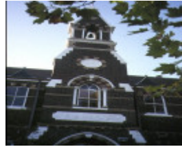
primary school number 1467 malvern road hawthorn detail of bell tower
