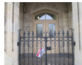
H0516 FORMER ES&A BANK (MANRESA PEOPLE'S CENTRE) LHA 2015 3.JPG
