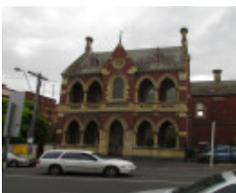
H0516 FORMER ES&A BANK (MANRESA PEOPLE'S CENTRE) LHA 2015 1.JPG
