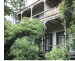
grace park house hawthorn front elevation
