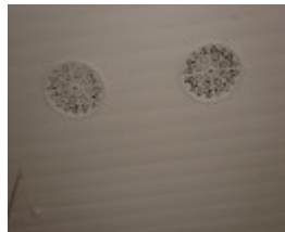
State school 2828 ventilators in ceiling KJ 26 Jul 07
