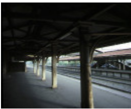
hawthorn railway station platform detail
