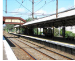
HAWTHORN RAILWAY STATION COMPLEX SOHE 2008
