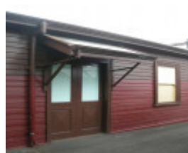
Platform 1 building - glazed timber doors and awning within the southeast-facing elevation
