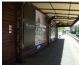
Looking south beneath the Platform 1 cantilever-truss canopy
