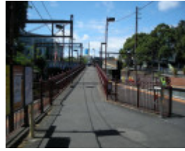
Looking north and upwards along the pedestrian walkway which links the island Platforms 2 and 3 with the south-side footpath on Burwood Rd bridge
