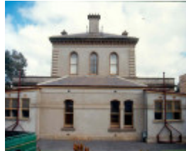
H01997 stawell courthouse rear sep01 ac2
