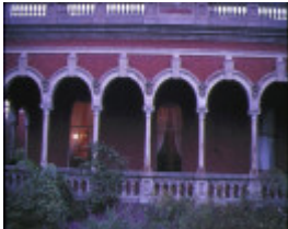
oxford isabella grove hawthorn arches along verandah
