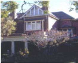
h00788 shenton kinkora rd hawthorn rear view
