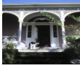
zetland yarra street hawthorn detail front entrance mar1987
