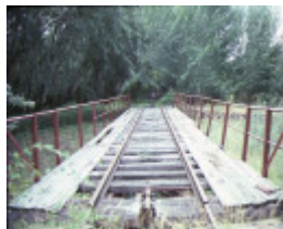
healesville railway station complex healesville kinglake road healesville tracks feb1985
