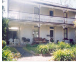
h00388 1 innisfail high street heathcote view from driveway she project 2003
