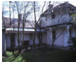
innisfail heathcote rear view aug1979
