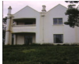
banyule heidelberg 1908 additions sep1995
