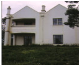
banyule heidelberg 1908 additions sep1995
