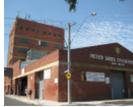
Hutchinson's Flour Mill (former) - 1-7 Marlborough Street (corner of Hartington Street), Glenroy
