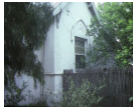
Former Head Teacher's Residence Heidelberg Side Windows September 1984
