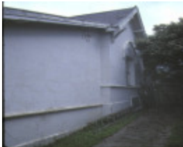
Former Head Teacher's Residence Heidelberg Side View September 1984
