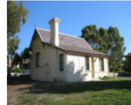
h01617 former head teacher's residence heidelberg side view 02 jan2001
