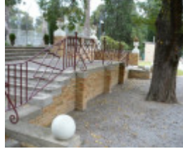
terrace adjacent to railway station
