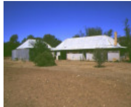
lake corrong homestead evelyn street hopetoun outbuildings
