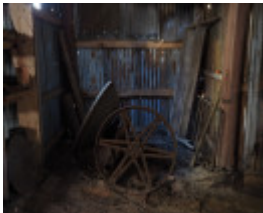
Battery House - Interior
