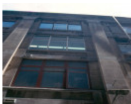
h01135 warehouses 2 3 oliver lane exterior detail 03 04 mz
