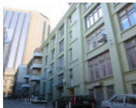
h01135 1 warehouses 2 3 oliver lane exterior 03 04 mz
