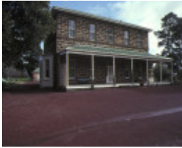
1 mt talbot homestead mt talbot horsham homestead front elevation sep1979
