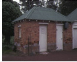
mt talbot homestead mt talbot horsham coldstore room
