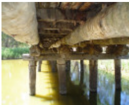
h01850 danns bridge over bet bet creek dunolly eddington road eddington underneath she project 2004
