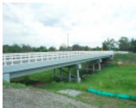
BAYLES BRIDGE NO.1 & 2 SOHE 2008
