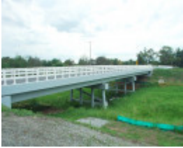
BAYLES BRIDGE NO.1 & 2 SOHE 2008
