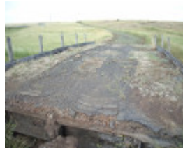
BURCHETT CREEK BRIDGE SOHE 2008
