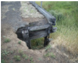
BURCHETT CREEK BRIDGE SOHE 2008
