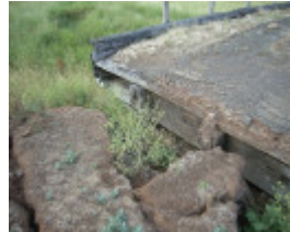
BURCHETT CREEK BRIDGE SOHE 2008
