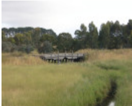
BURCHETT CREEK BRIDGE SOHE 2008
