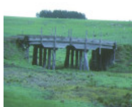
1 burchett creek bridge ntv
