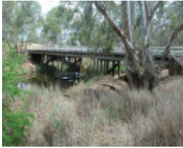
FERGUSONS BRIDGE SOHE 2008
