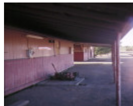
irymples railway station irymple avenue irymple platform verandah
