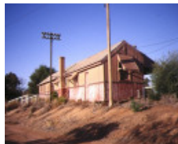
irymples railway station irymple avenue irymple rear view apr1995
