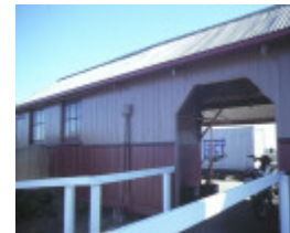
irymple railway station irymple avenue irymple entrance aug1984
