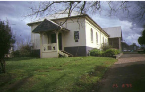
1 st stephens church and school portland
